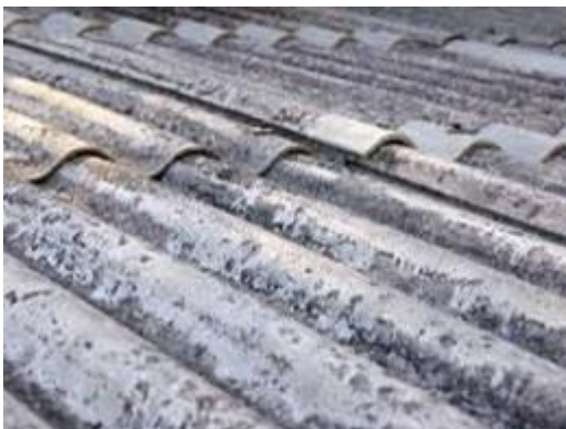
Asbestos cement roof
