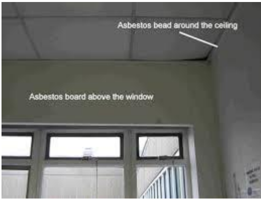
Asbestos panelling
